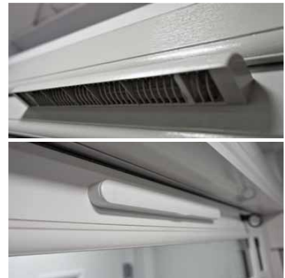
Trickle Vents Adjustable internal tumbler and external built in fly screen.
